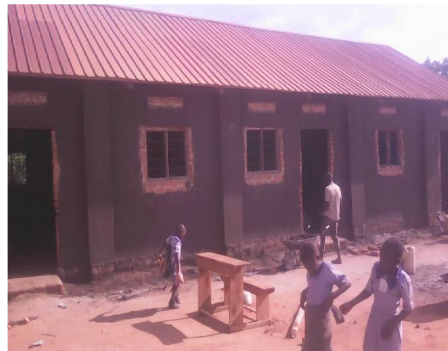
External plastering done
