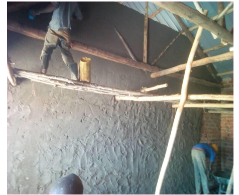
Plastering the Partition
