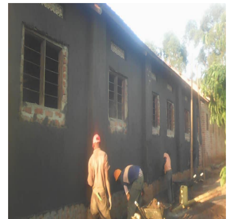
Plastering the Partition
