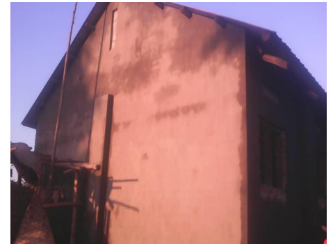
Pin wall plastered
