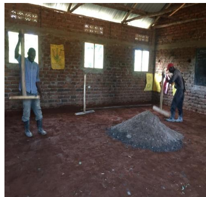
Making and Cementing Concrete Floors
