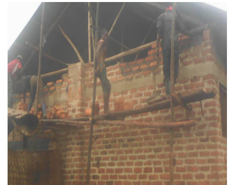
Collapsed Shade under Repair
