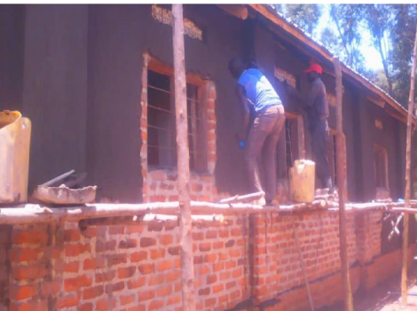
Plastering in progress
